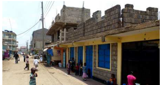
Komarock - suburb in Nairobi. Houses are being built brick by brick depending on the available finances
